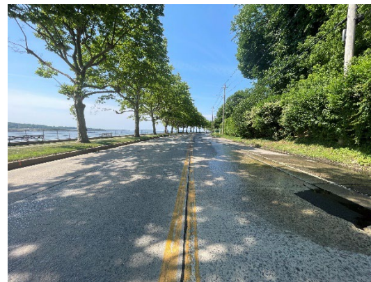
Exposed concrete panels
